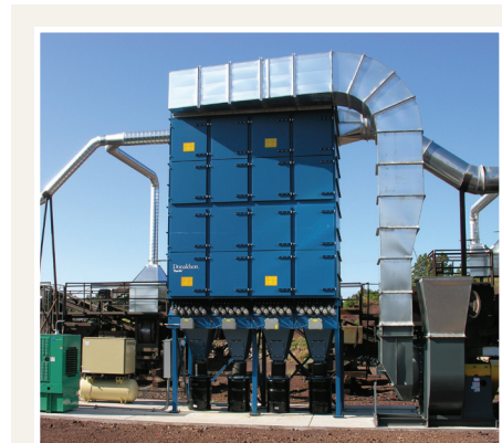
DALAMATIC® DUST COLLECTOR
